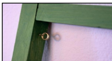
STEP 1 - Insert D-rings or screw-eyes into frame
